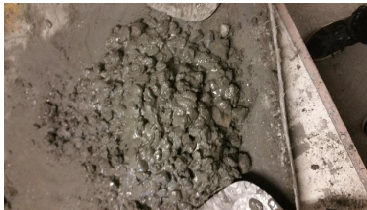
Figure 3.3 Mixing of Concrete.
