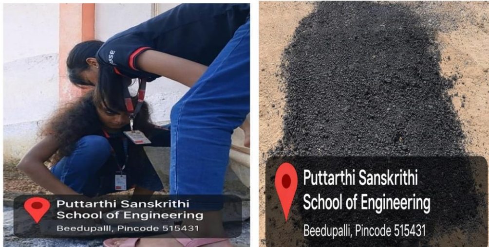
Figure.1. flexible pavement with partial replacement of bitumen with plastic.
