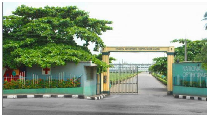
Figure 1: View of the Major hospital complex, national orthopedic hospital, Lagos.
